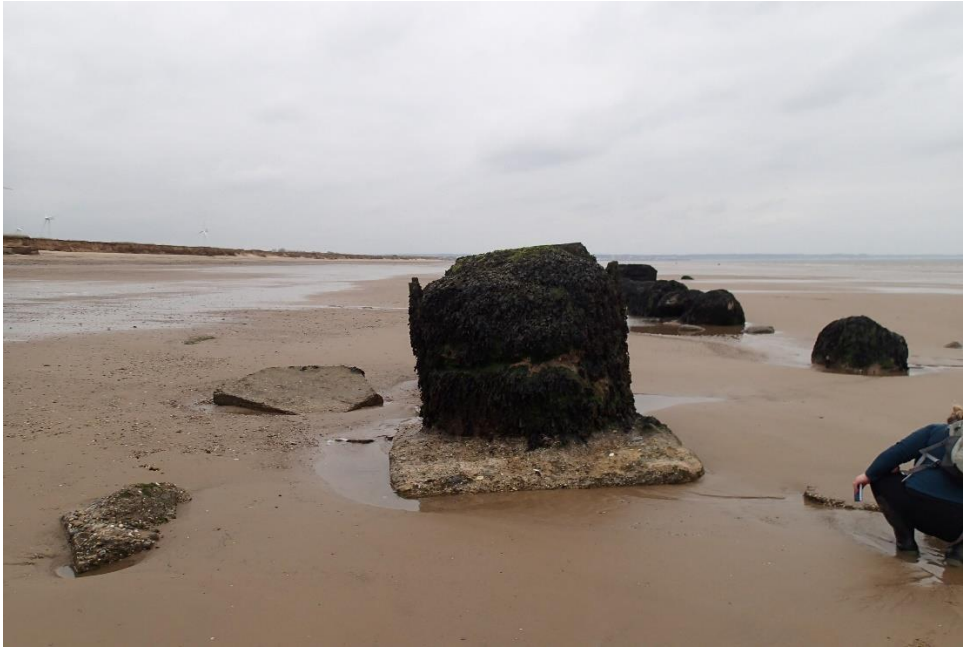
Plate 8. Eroded war time coastal fortifications with attached algae and scour pools. T3 mid-shore (site ref 281).
